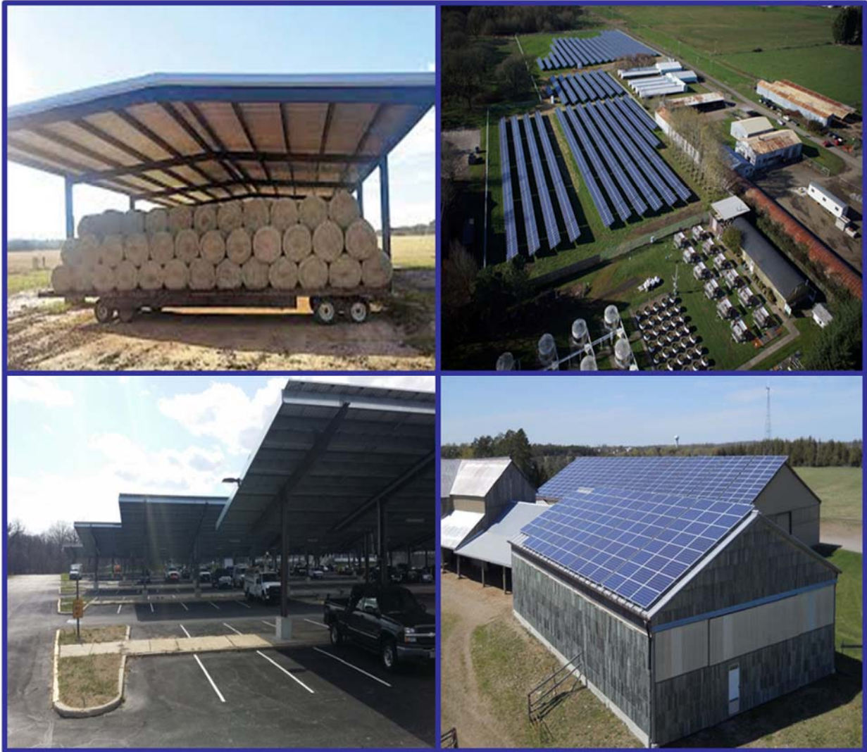
Figure 4: Examples of proposed types of solar facilities at BARC
